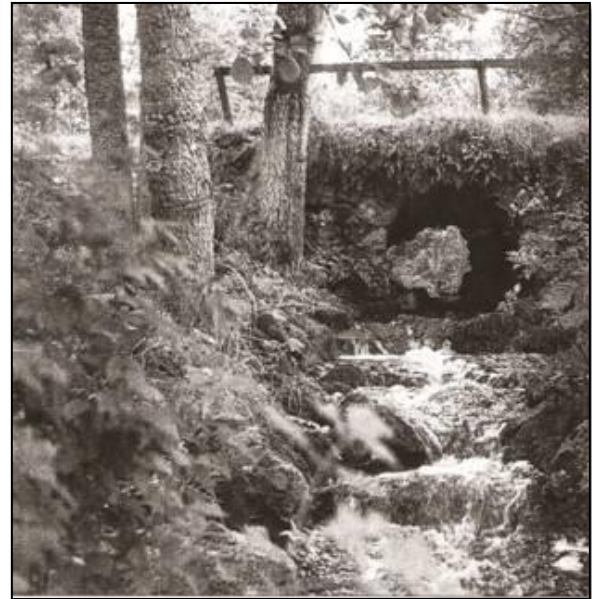
Old bridge at Broddarp
