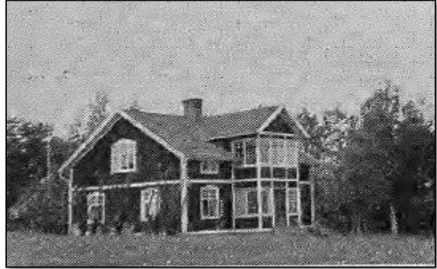
House at Rickelstorp
