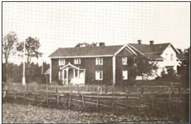
This house at Skattegården, Gransäng was originally built in 1751 and was originally much
