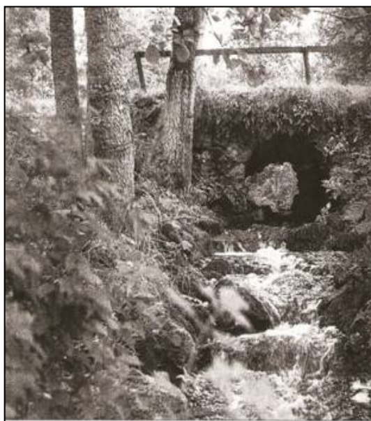
Old bridge at Broddarp
