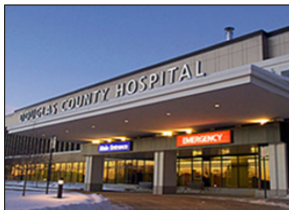
Douglas County Hospital – Alexandria, MN
